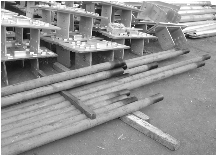
Steel parts to be inserted on ground before erection
