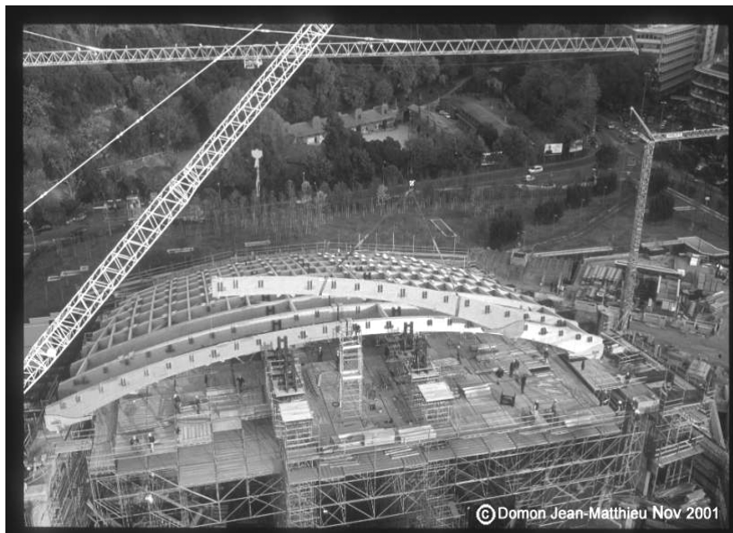
The 18 trusses of hall 2700 are lifted with a 400 TONS crane
