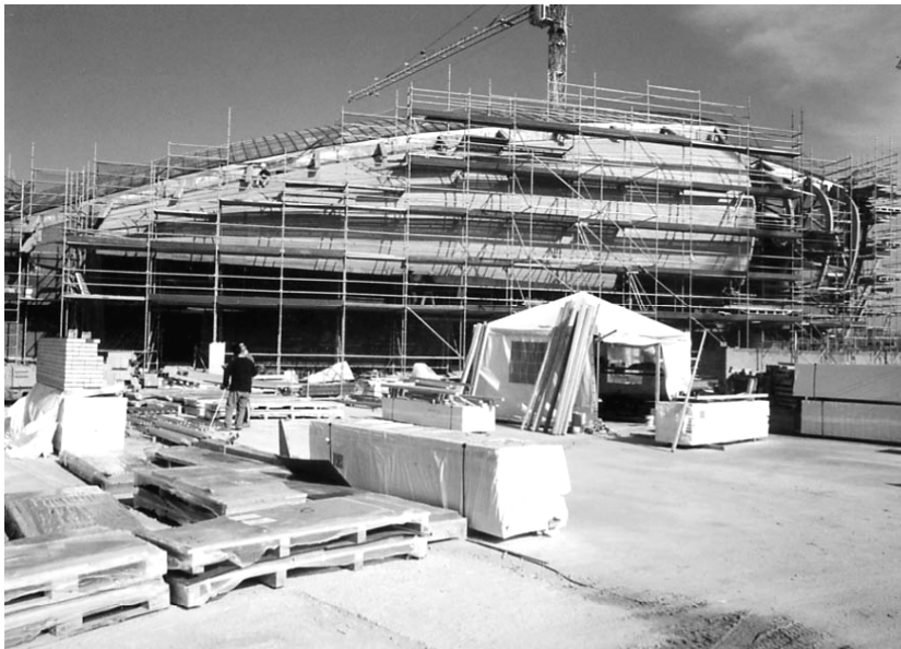
Storing area of steel and glulam materials
