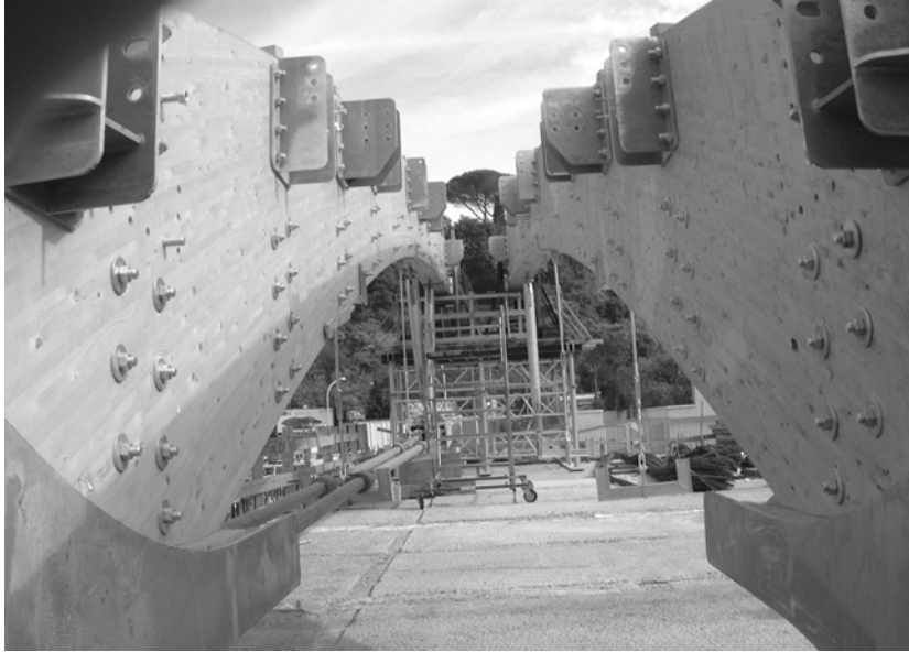
Two half beams, before erection
