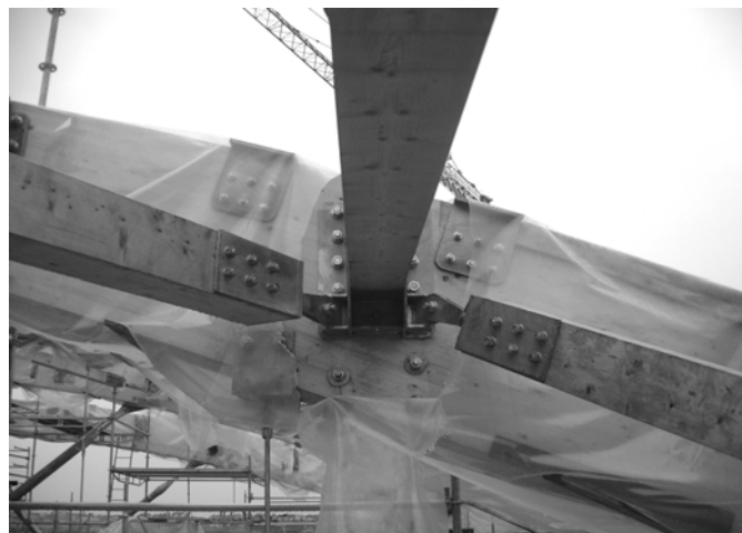
Glulam Wind bracing
