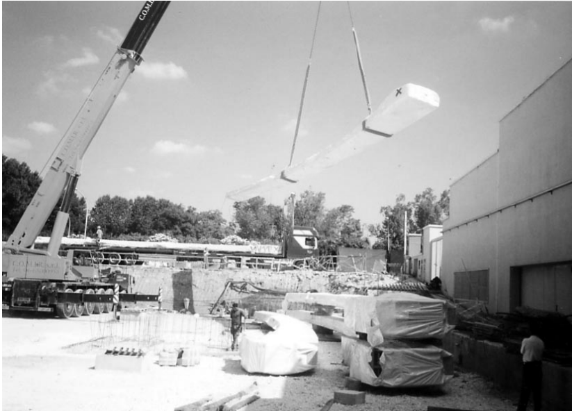
Unloading half-arches : max tot weight: kg. 14.700 hall 2700 type G10-G11.
