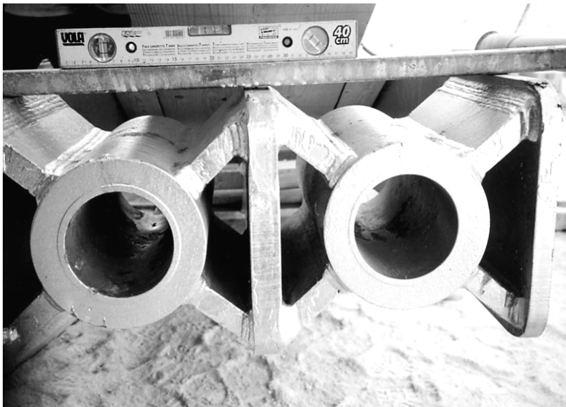
Assembling the twin traction rods: diameter 100mm (hall 2700)
