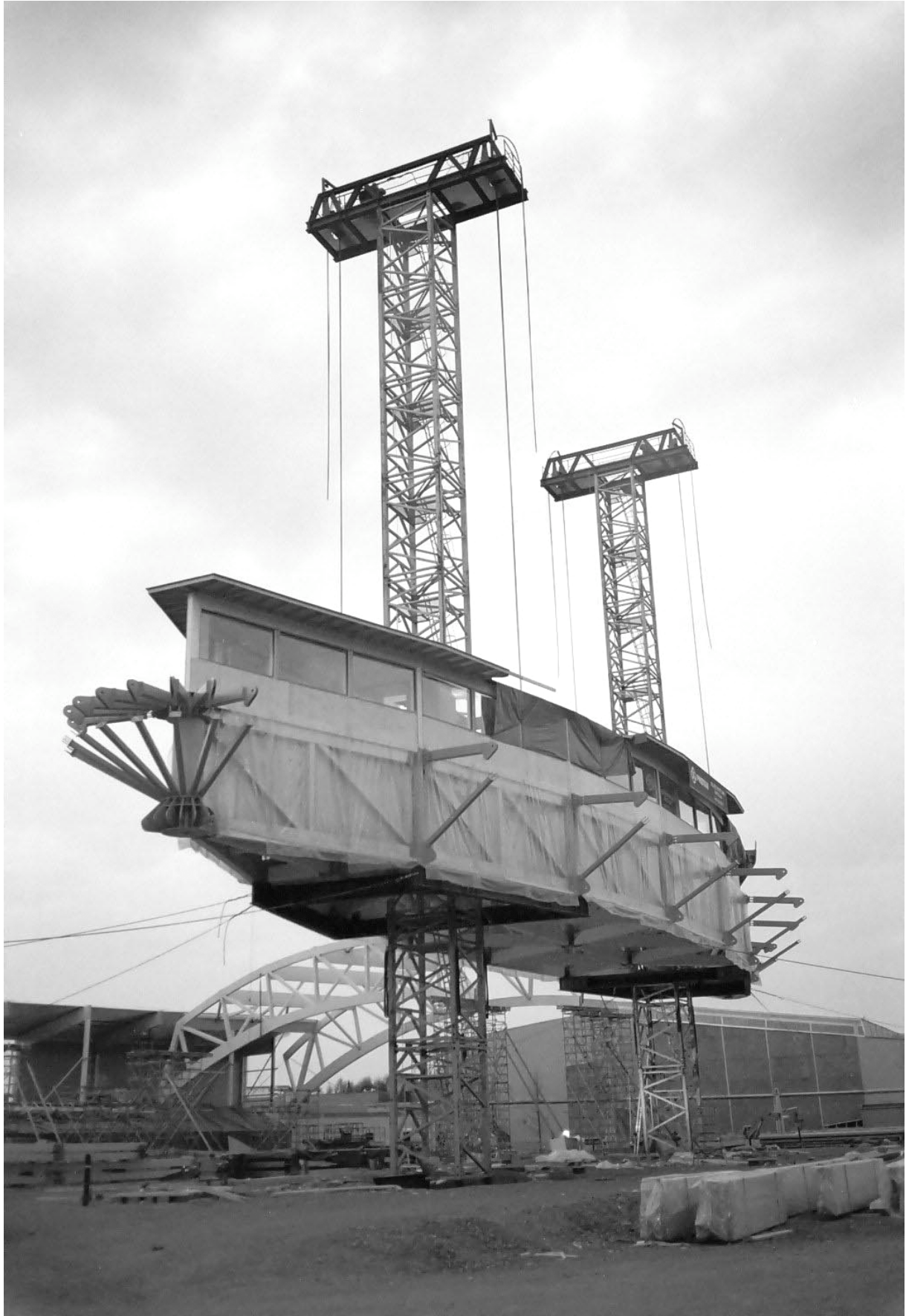
Picture 6: Hoisting of the space truss with four hydraulic jacks
