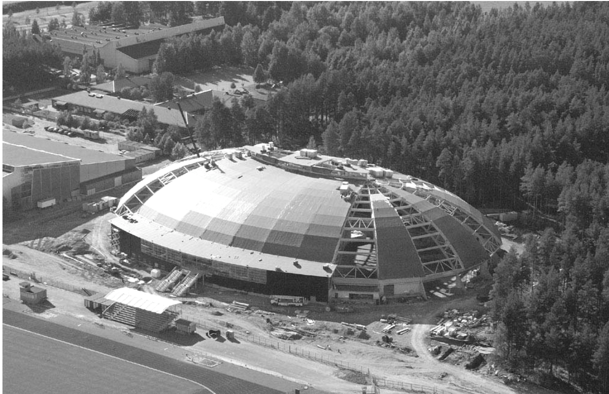
Picture 1: The Joensuu Hall under construction in the autumn of 2003
