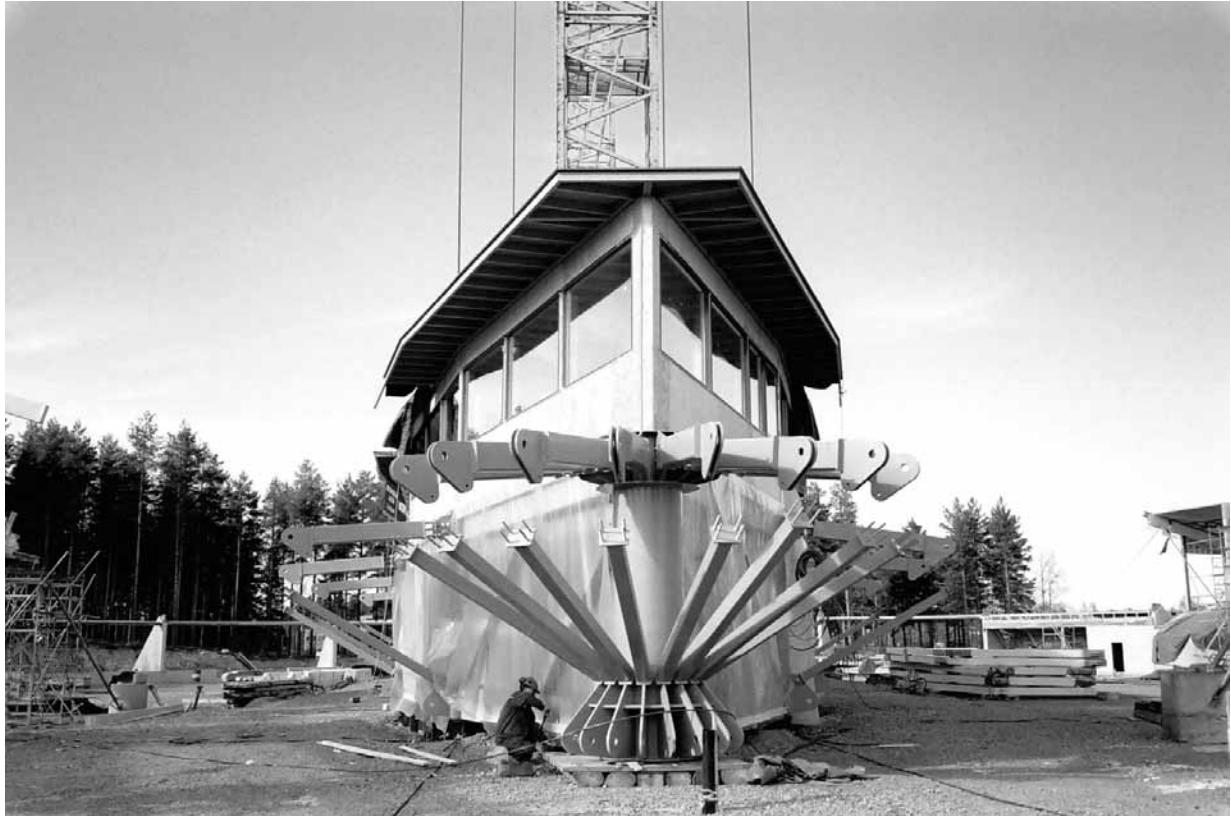
Picture 4: Installation of the space truss
