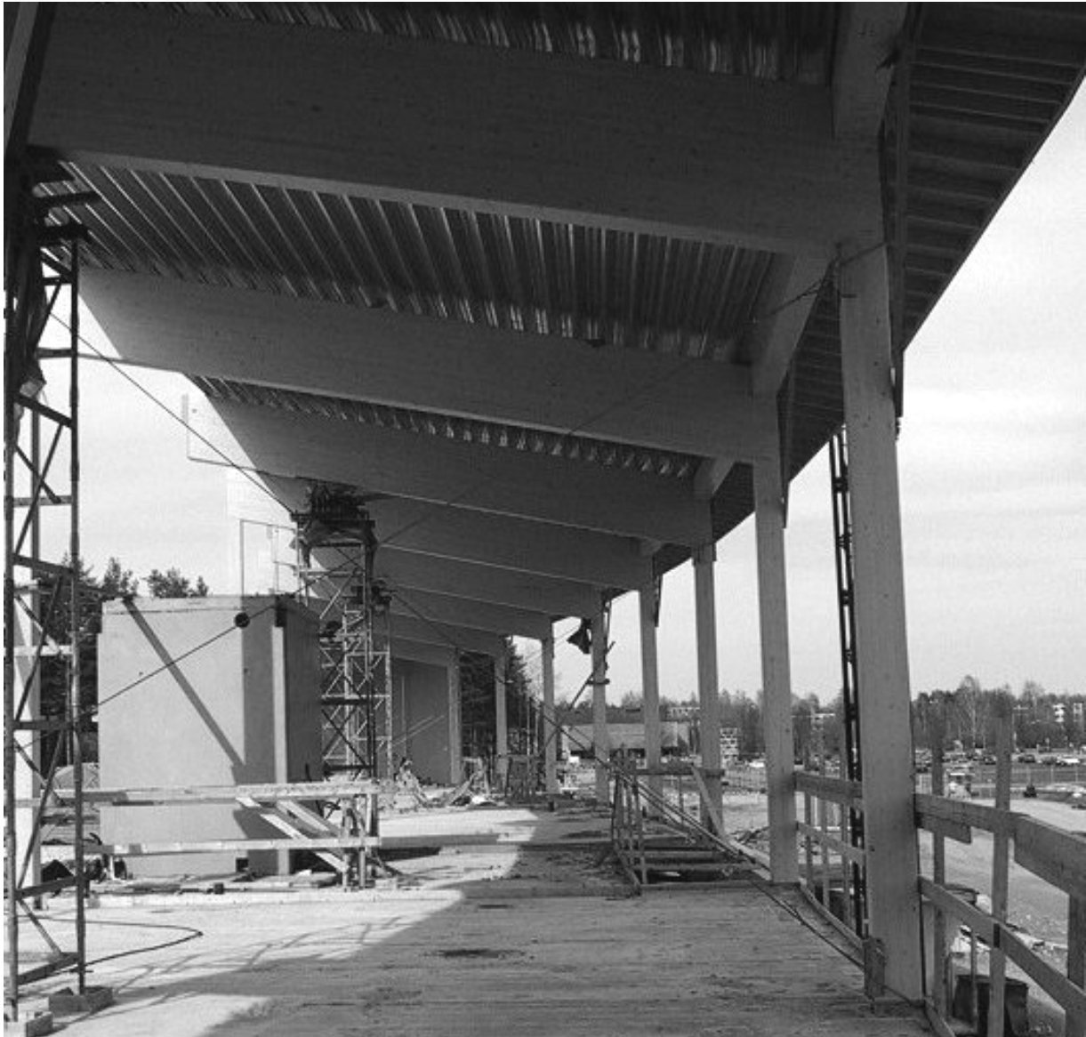
Picture 3: Installation of the wood frame of the service premises
