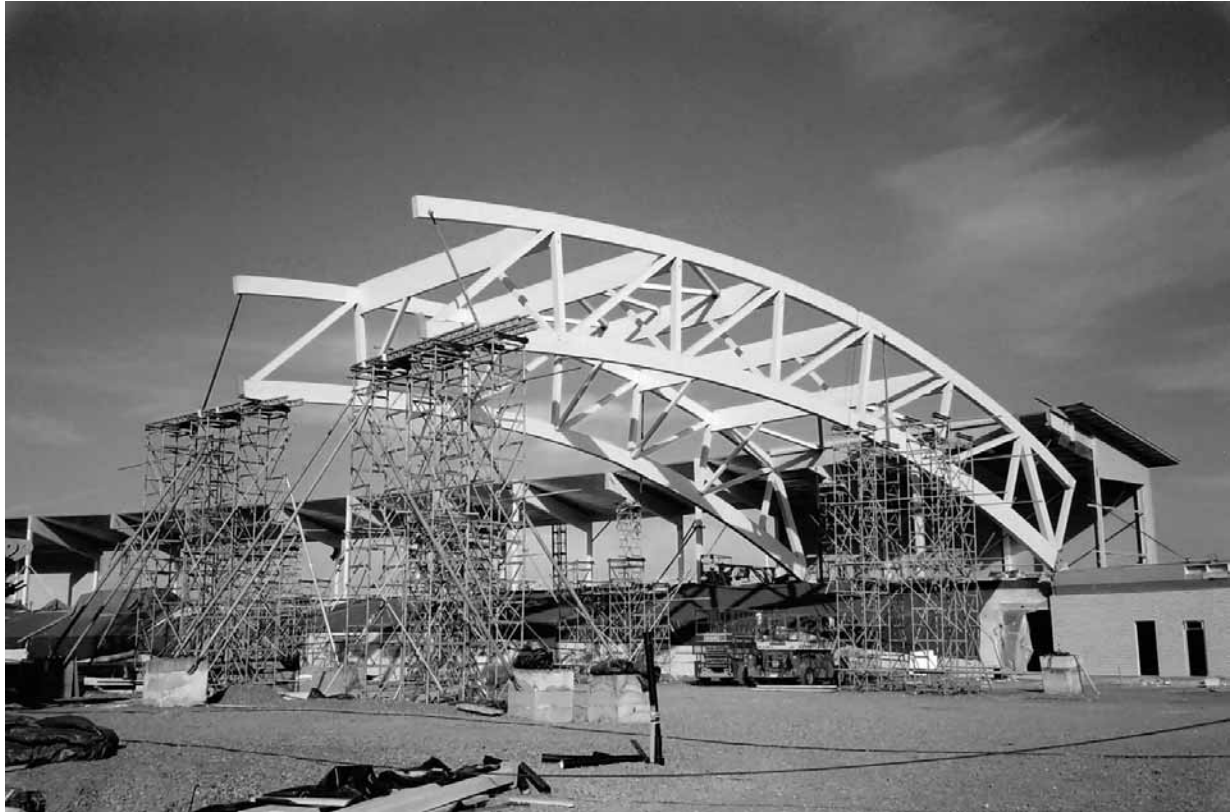
Picture 7: Installation of the main arc sections
