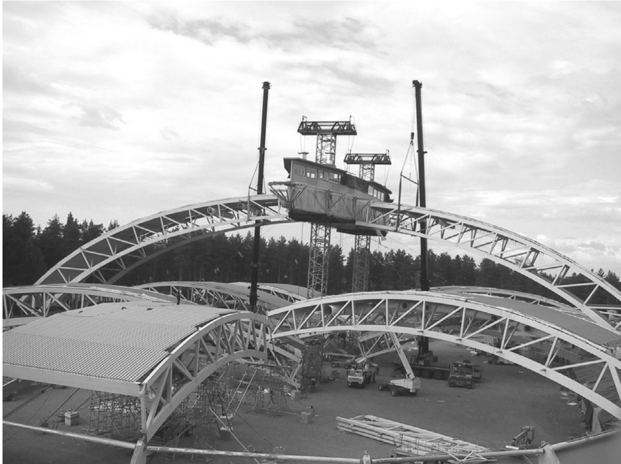
Picture 8: Hoisting of the main arc sections with mobile cranes
