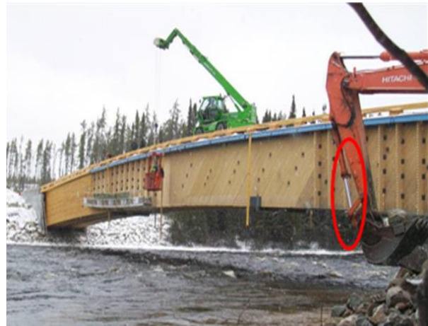
Image 23: Installation of the exterior siding to protect against the elements
