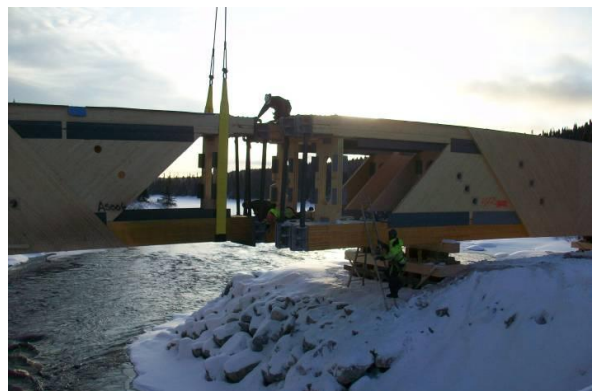
Image 22: Installation of the individual elements in extreme winter conditions
