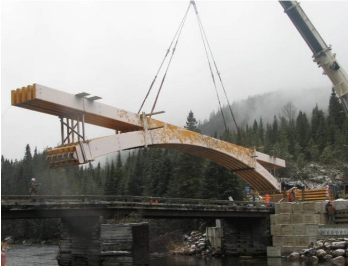
Image 13: Montmorency bridge (38,4m length, 32,5m free-span, 175 tonnes capacity)
