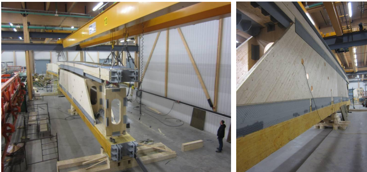
Image 20: Prefabrication in the factory
