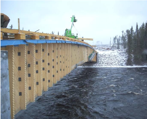
Image 23: Installation of the exterior siding to protect against the elements
