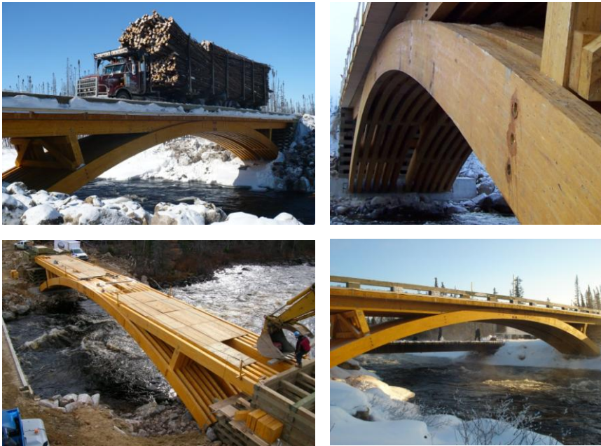
Image 11: Témiscamie bridge (41,9m length, 34,9m free span, 175 tonnes capacity)
