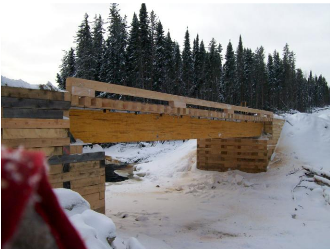
Image 15: Barette-Chapais bridge (4,6 m wide, 17m free-span, 175 tonnes capacity)
