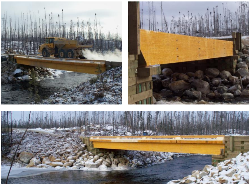
Image 12: Petite Témiscamie bridge (4,6m wide, 21,4m free-span, 175 tonnes capacity)
