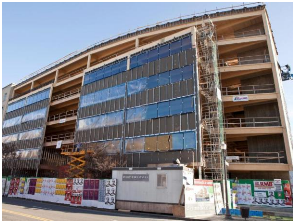
Image 8: Multi-storey office building in Quebec City, QC
