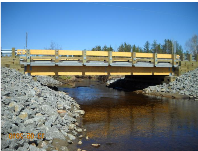
Image 14: Albabel bridge (7,3m wide, 11,6m free-span, 175 tonnes capacity)
