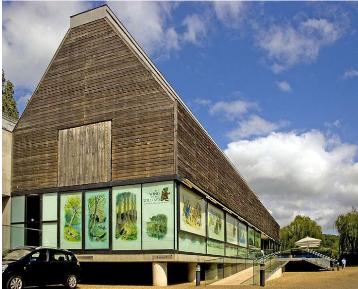
The River and Rowing Museum in Henley-on-Thames, Oxfordshire by David Chipperfield Architects
