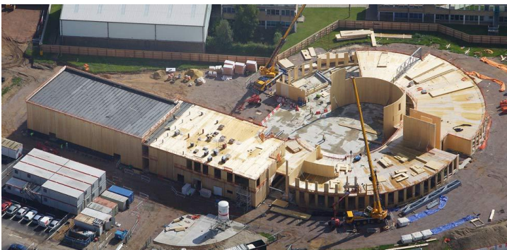
Open Academy Norwich under construction
