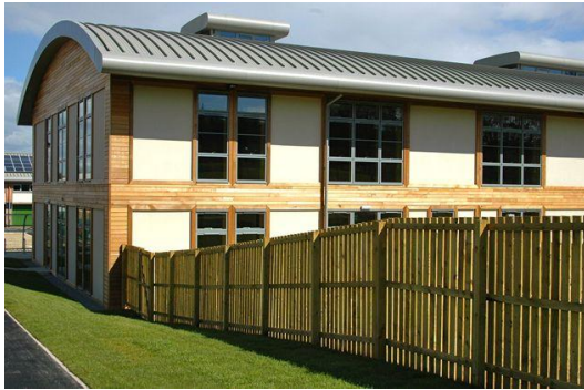
Illustration 3: Prefabricated straw bale panel system Inspire Bradford Business Park. Image copyright ModCell®
