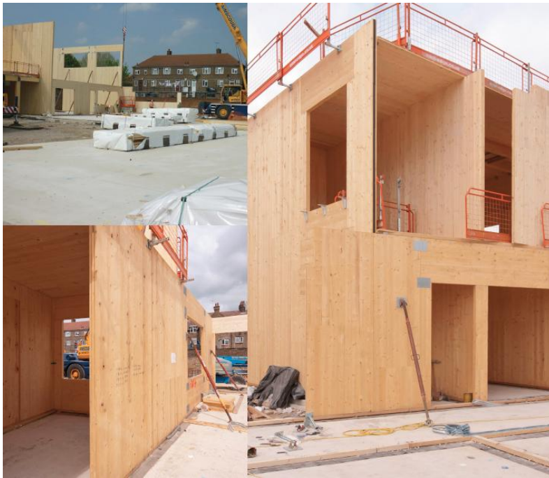
Illustration 7: Manor Longbridge primary school under construction. Image copyright X-Lam Alliance
