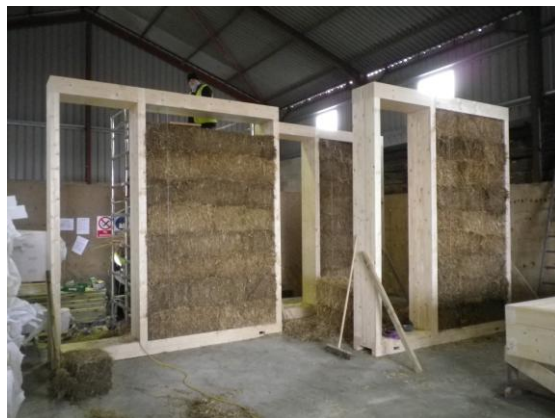
Illustration 4: Prefabrication for BaleHaus® test building and completed building. Photo U of Bath
