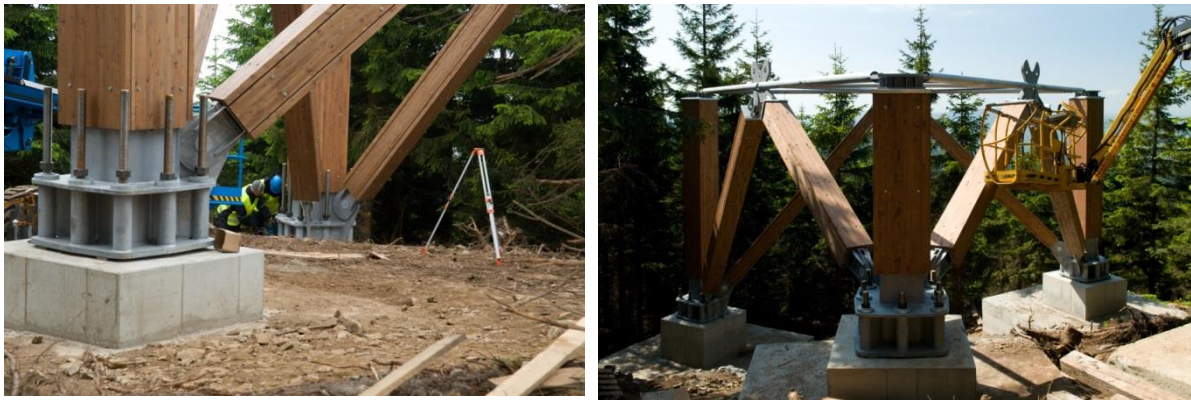
Figure 7: Anchoring of columns of main load-bearing structure
