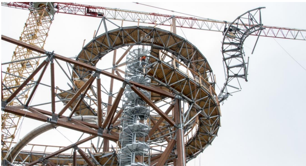
Figure 8: Assembly of main load-bearing structure of the footbridges
